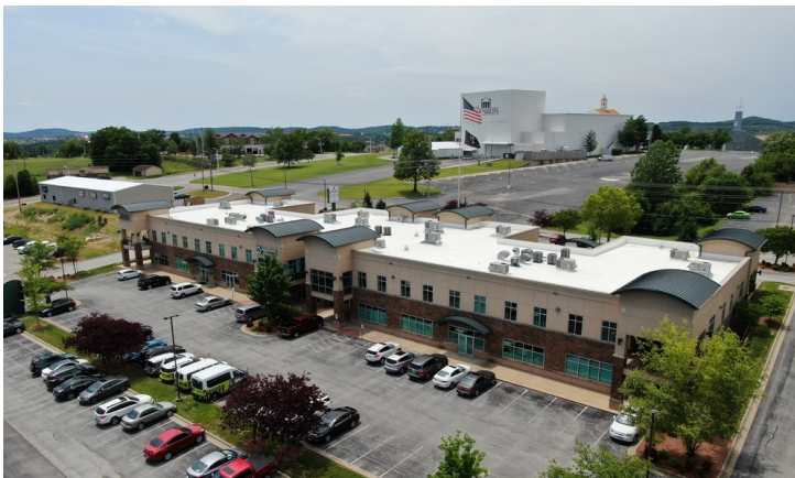
Rear View Looking South West
