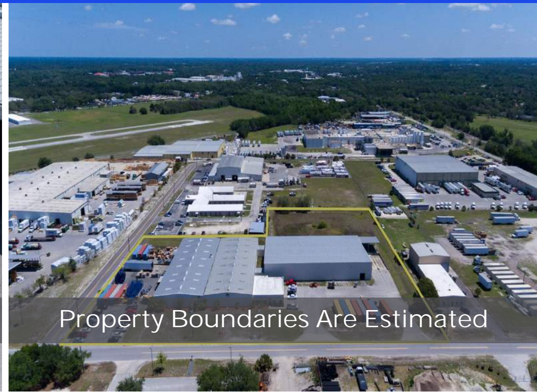
Northside Docks and Grade Level Loading
