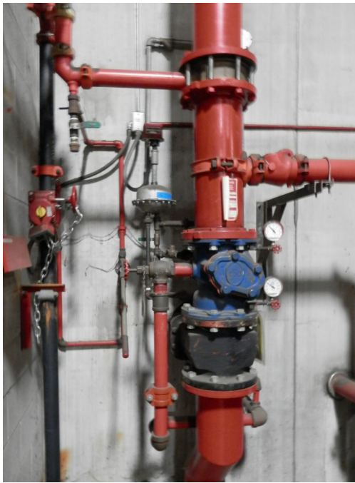
Fire Suppression System for Racking
