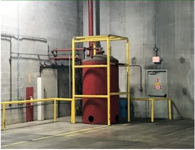
Fire Suppression System for Racking
